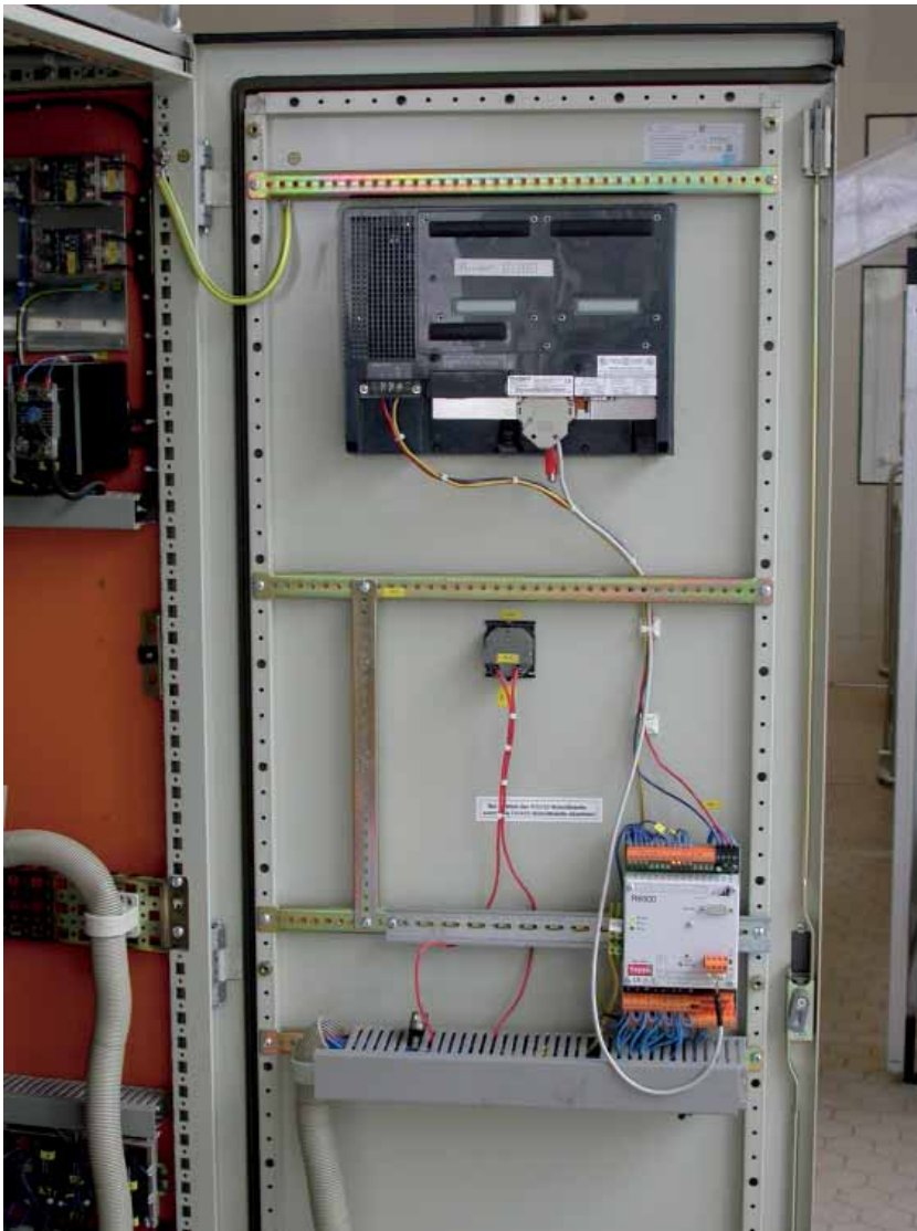
Stand-Alone Solution: Autonomous R6000 Controller and Control Terminal
